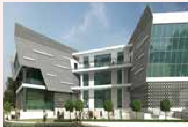
Work started in 2018, completion by end of 2020
