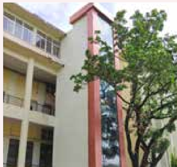
Installation of new Lift in Physiology Block -KMC
