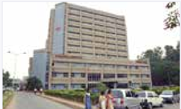
Manipal Hospital, Bengaluru
